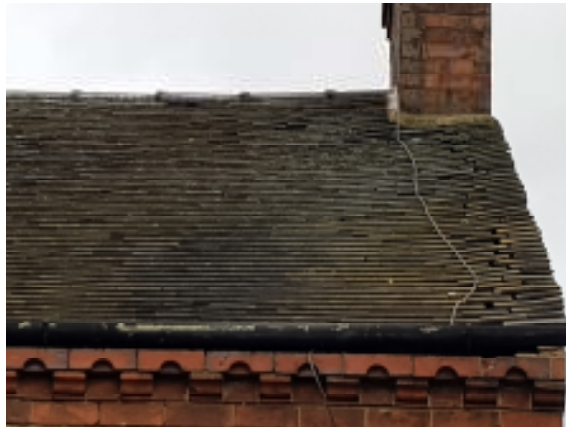
Plate 6: Showing raised roofing tiles.
