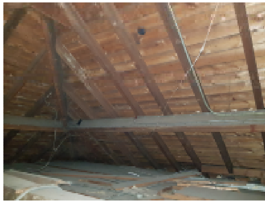
Plate 11: Showing internal view of roof void
