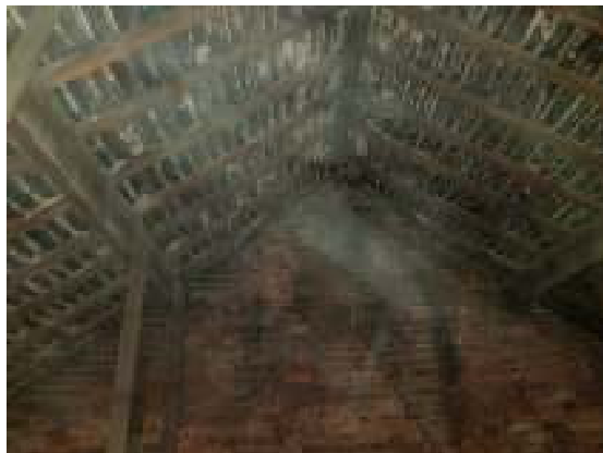
Plate 7: Showing internal view of roof void
